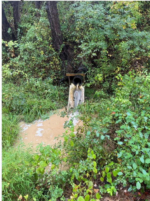
Figure 6: Culvert creating WOTUS 2, directly above northern section of racetrack
